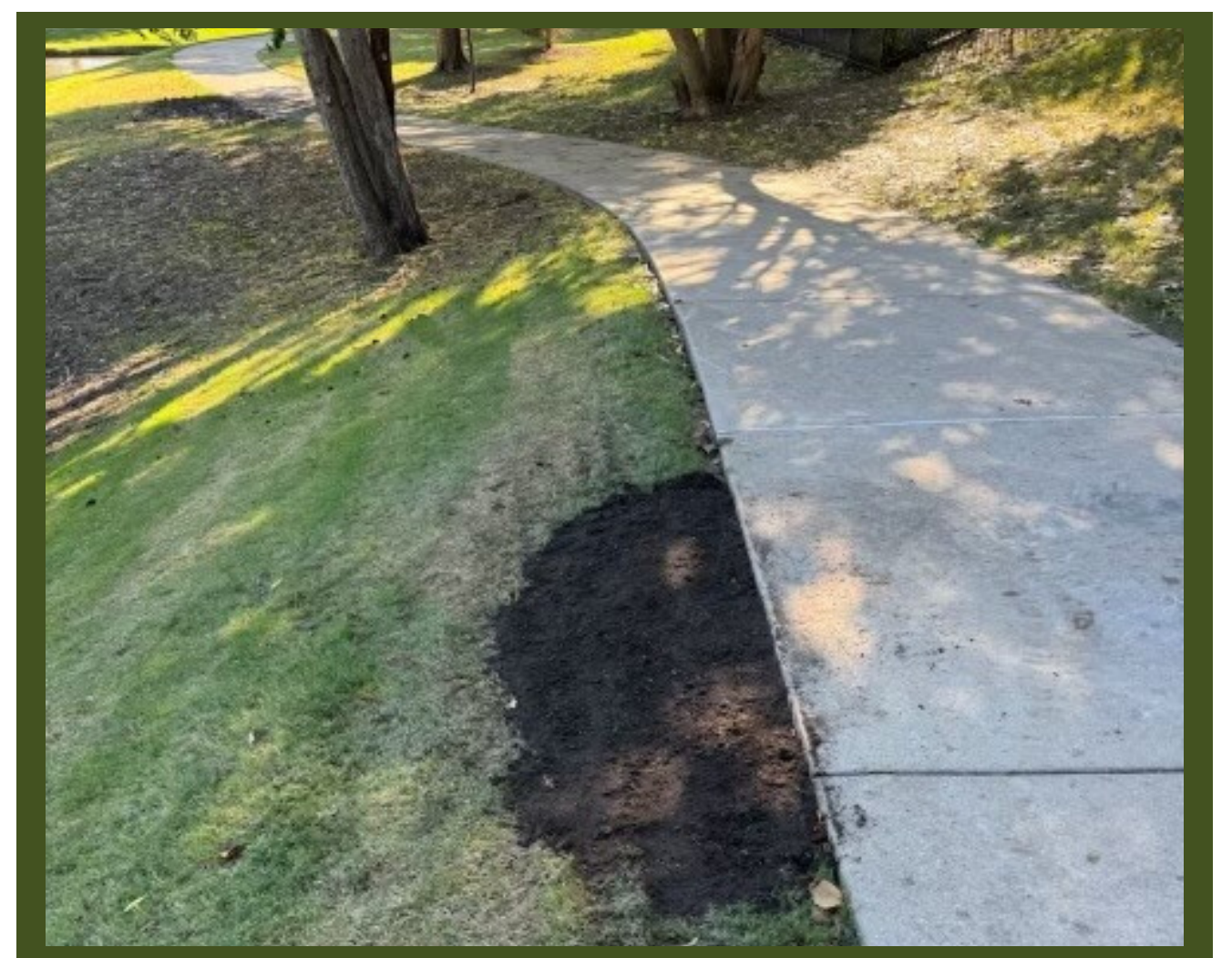
EMERALD BAY SINK HOLE REPAIR AFTER
